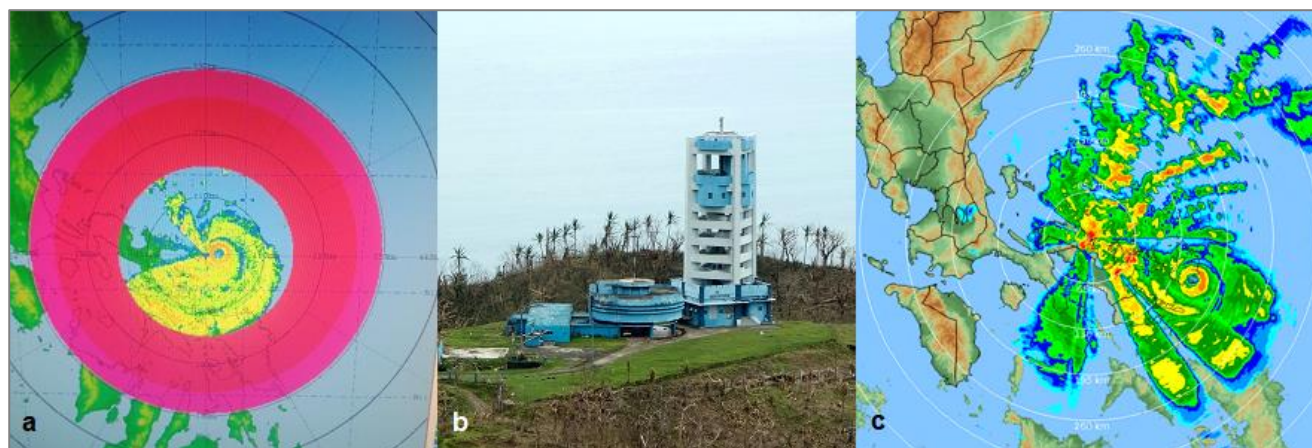
Figure 26: The last known observation (2030 UTC on 31 October 2020) from Bato weather radar (left). The pink circular band is an indication of the impending failure of the radar antenna. The post-storm aerial survey over the PAGASA weather radar in Bato, Catanduanes, where the pedestal of the radar antenna can still be seen standing on the tower rooftop (centre). The reflectivity image from Daet weather radar when Typhoon Goni (Rolly) made landfall over Bato, Catanduanes, at 2050 UTC on 31 October 2020 (right).
